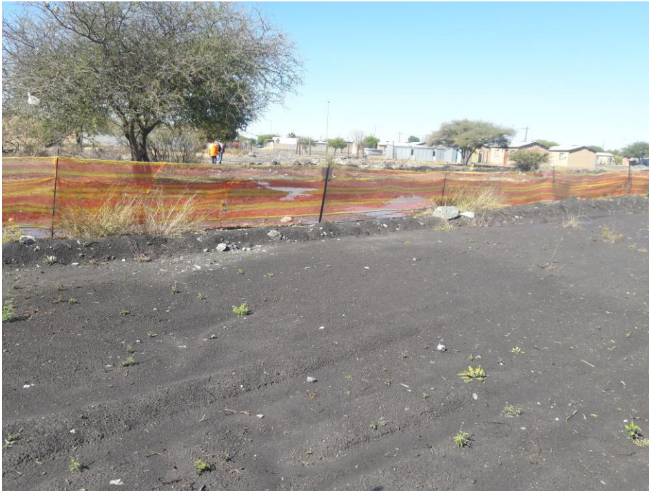
Photo 3: Storm water diversion berm diverting storm water away from substation site
